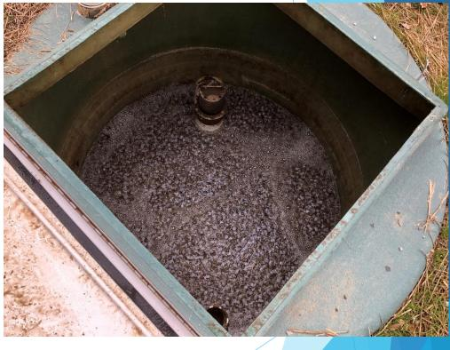
New System ~ Trickling Filter (effluent polishing)
