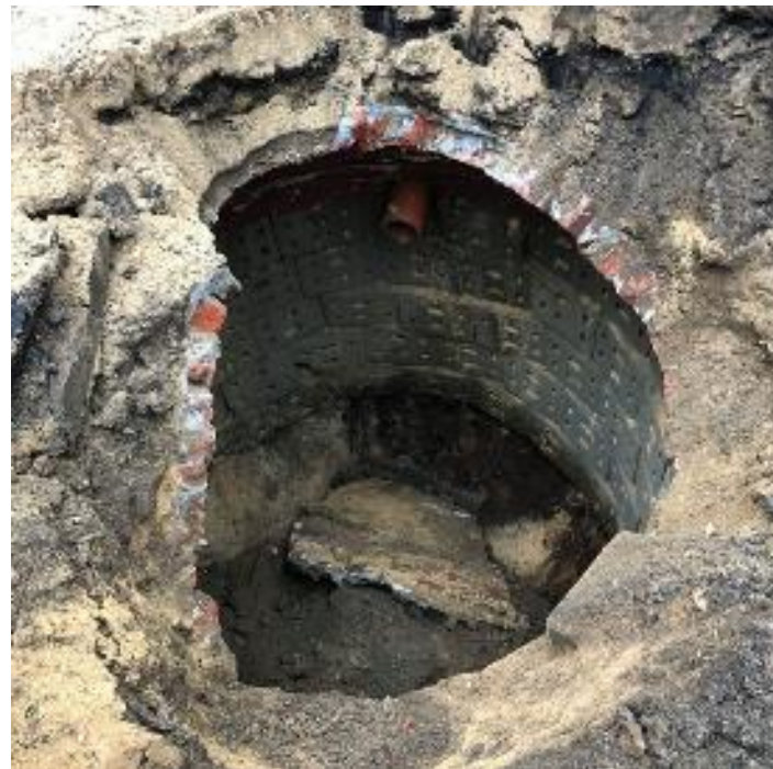
Collapsed Cesspool
