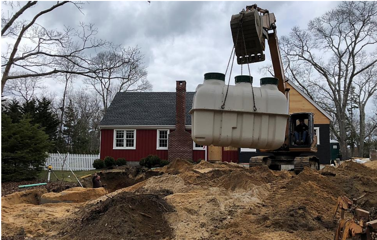
Fuji Clean IA Septic System During Installation
