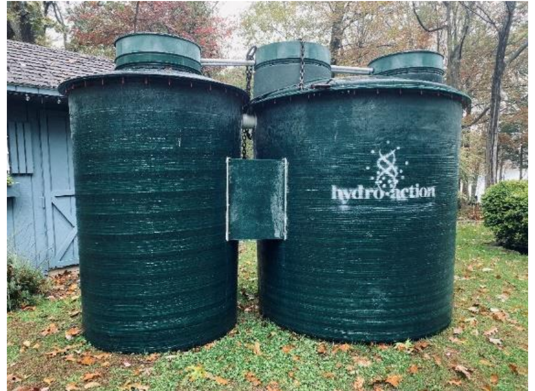
Hydro-Action IA Septic System Prior to Installation
