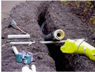
Trencher to dig 2-3 feet deep; insulated line for cold climates (on right). Or directional boring. Source: Siegrist, 2017
