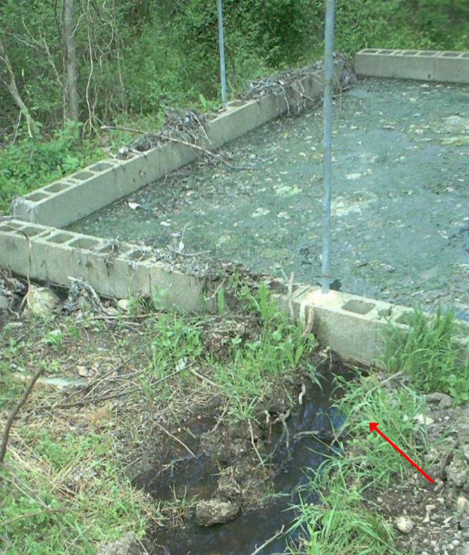
Lagoon serving restaurant leaking through southwest side of wall at left, and block removed allowing discharge at right.
