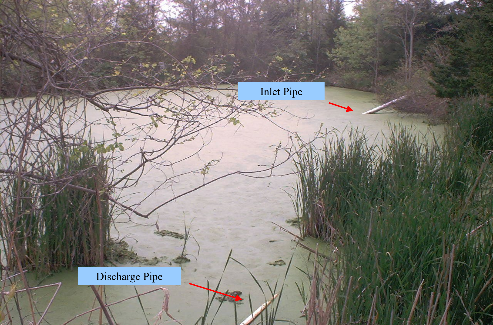
Single cell lagoon serving a resort on Table Rock Lake manager's residence and three adjoining rentals. White pipe in upper right of photo is inflow pipe, smaller pipe at lower center is discharge pipe that leads through lagoon berm.
