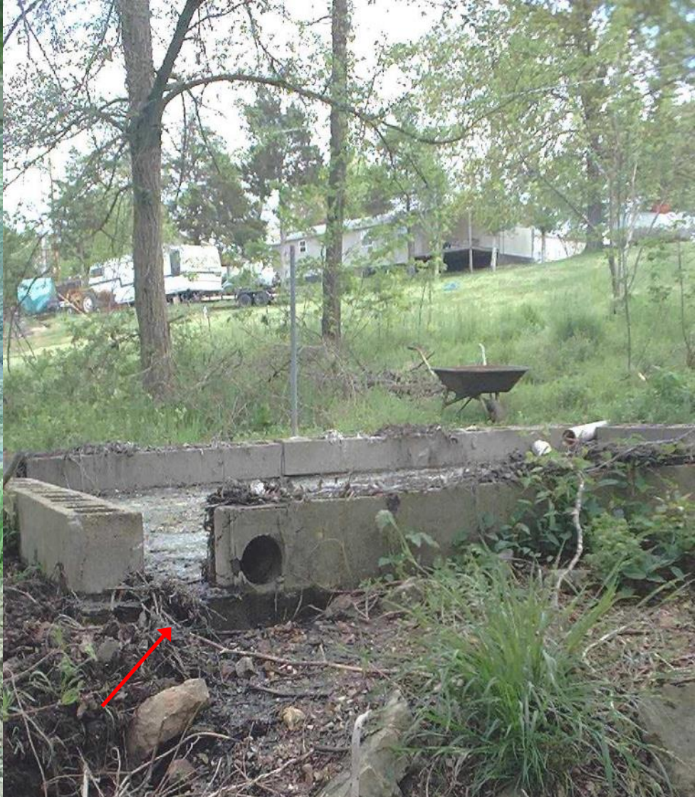
Lagoon serving restaurant leaking through southwest side of wall at left, and block removed allowing discharge at right.
