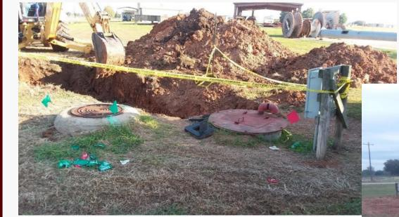
Connecting the Center with the RELLIS Sewer Main instead of just one building.... Original flow to the Center was <200 GPD!
