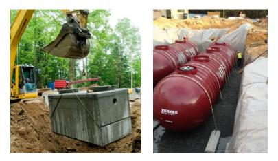
Must be designed and installed for H-20 load
