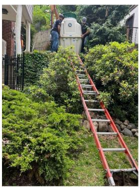
Figure 6. Installing a FujiClean Unit on Difficult to Access Site
