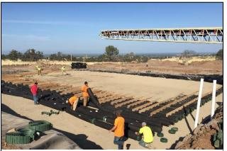
Fig. 5 – FEMA work camp wastewater treatment system
