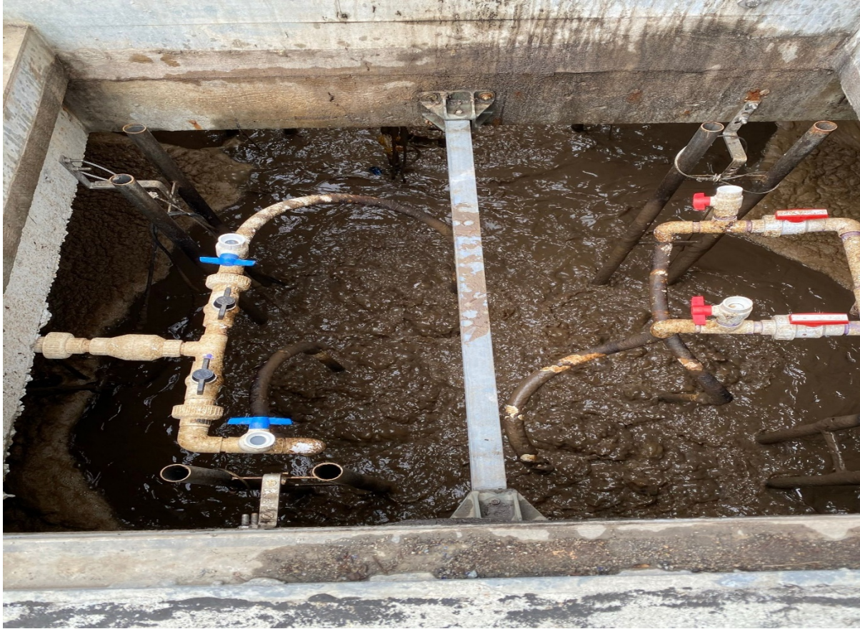
Figure 12. Coarse bubble aeration of HSMBR with \sim 10,000 mg/L MLSS
