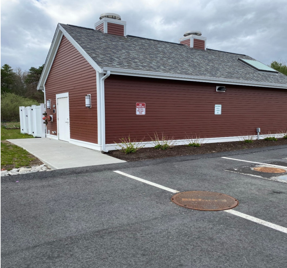
Figure 14. Sewage control house
