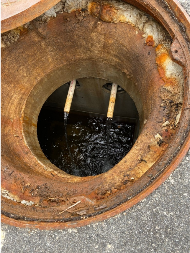
Figure 18. Permeate discharging to drip dose tank
