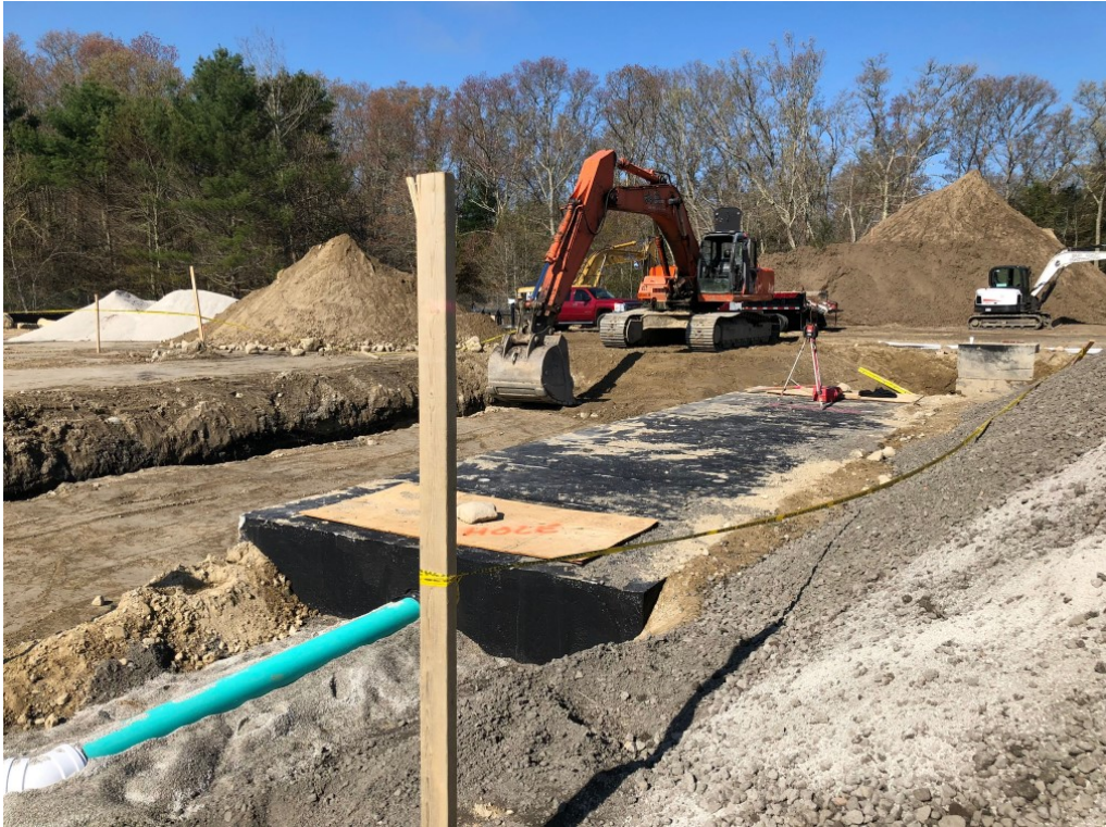
Figure 6. 20,000-gallon cast in-place tank installation
