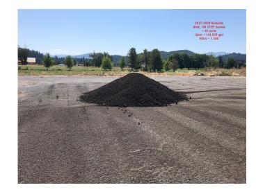
Two years of biosolids (20 cubic yards) for over 1000 connections in Glide, Oregon, naturally dried in a drying bed.
