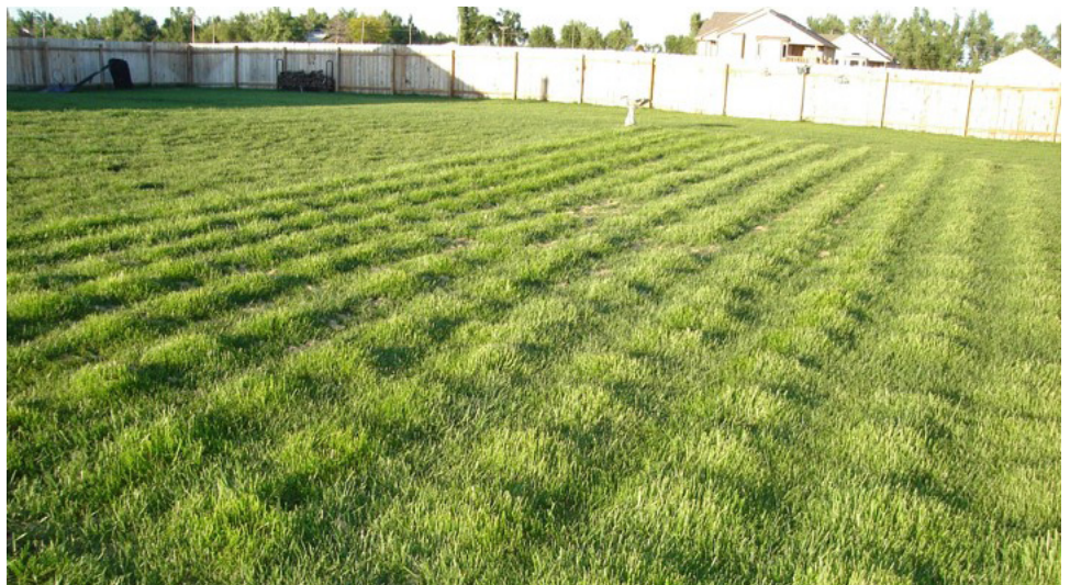
Photo 1. Uniform distribution of effluent over the entire dispersal area.
