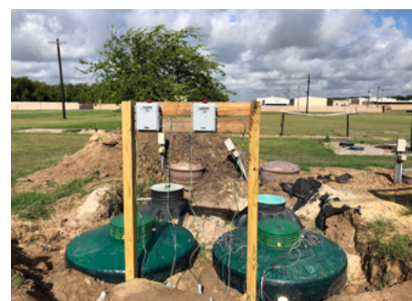
Photo 3. Tapping into the REL-LIS Campus sewer main to supply OSSF Research Center with raw wastewater.
