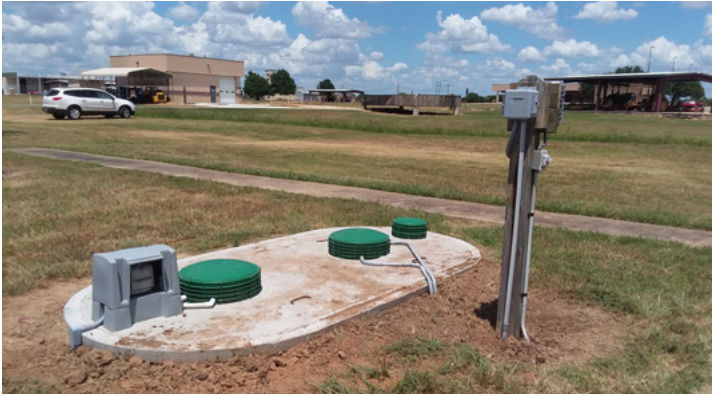
Photo 6. Reuse technologies, one with a membrane filter (BioMicrobics MBR0.5, shown on the right), and one without a membrane filter (Clearstream 500DA, shown on the left).
