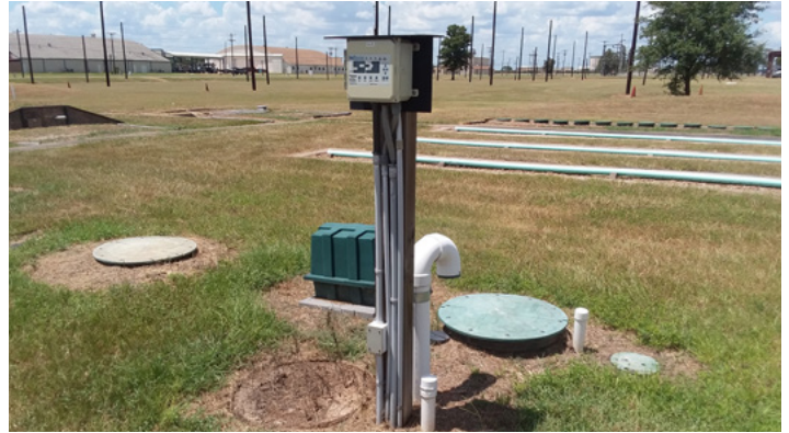
Photo 6. Reuse technologies, one with a membrane filter (BioMicrobics MBR0.5, shown on the right), and one without a membrane filter (Clearstream 500DA, shown on the left).
