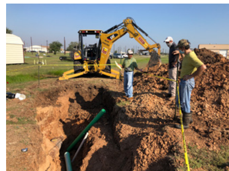
Photo 3. Tapping into the REL-LIS Campus sewer main to supply OSSF Research Center with raw wastewater.
