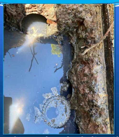
Crushed and overloaded distribution box
