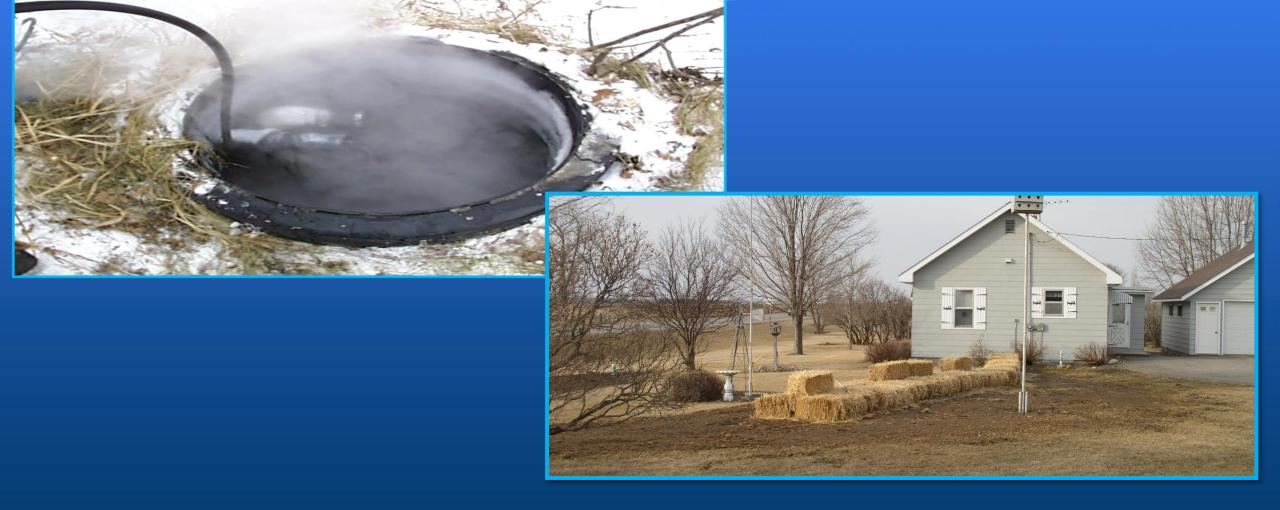
Frozen system and straw bales for insulation not removed
