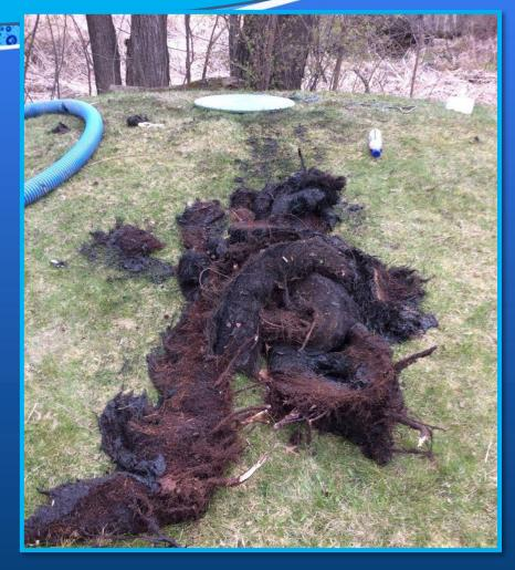
Roots in a distribution box and out of a septic tank
