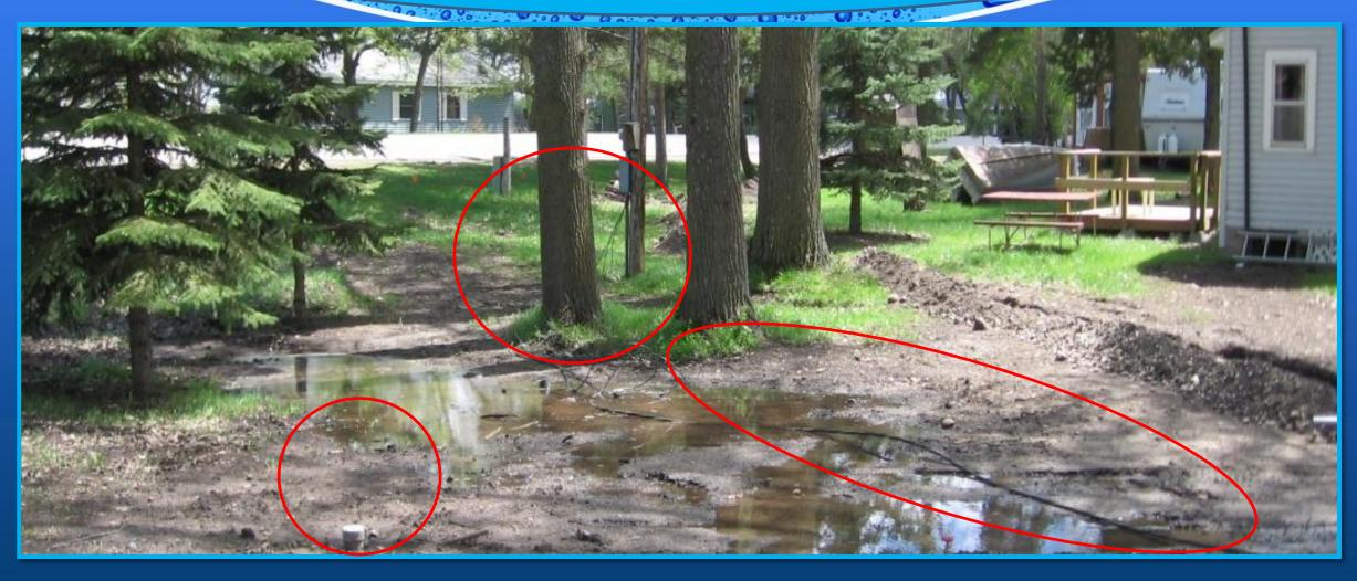
Electrical cord running through surface water to pump and poor surface drainage
