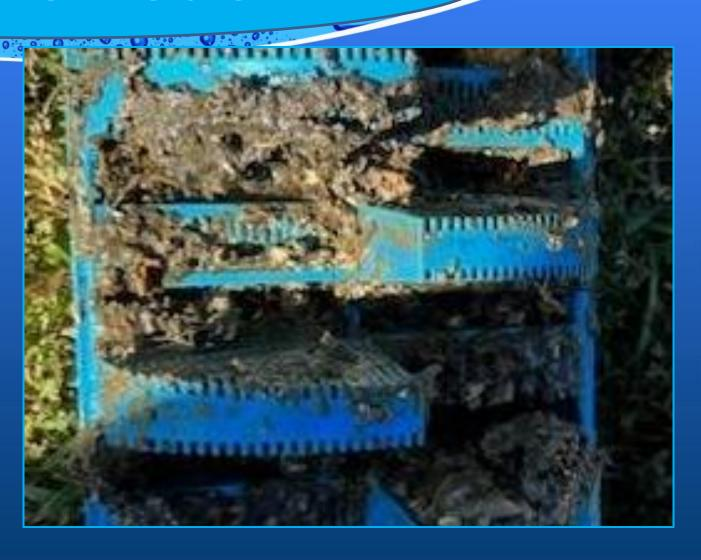
Plugged up effluent screen
