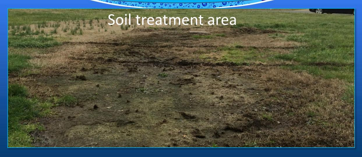
Surfacing of effluent and traffic over the system
