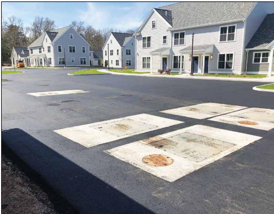
Photo 2: Treatment units safely installed underground in roadways but with easy maintenance access
