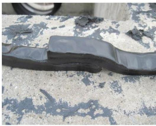
Figure 3 – Overlap of Butyl Sealant
