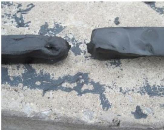
Figure 2 – Gap in Joint Sealant Application
