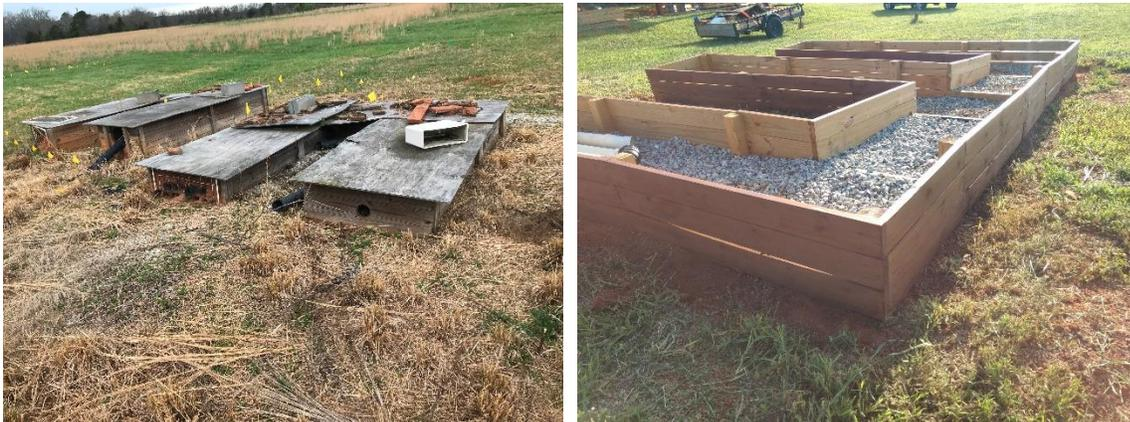
Figure 3. a) original serial box for individual approved products in Georgia which were deteriorated by the weather and removed, b) newly constructed serial box to be used for all approved products in Georgia. (Photos taken by E. Lunsford and G. Hawkins, 2019)
