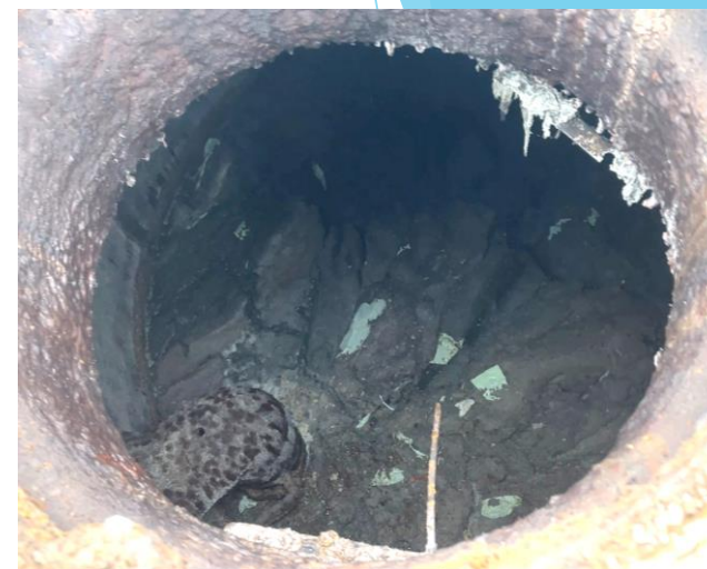
Before IMET Installation - Feb 25 th 2025
