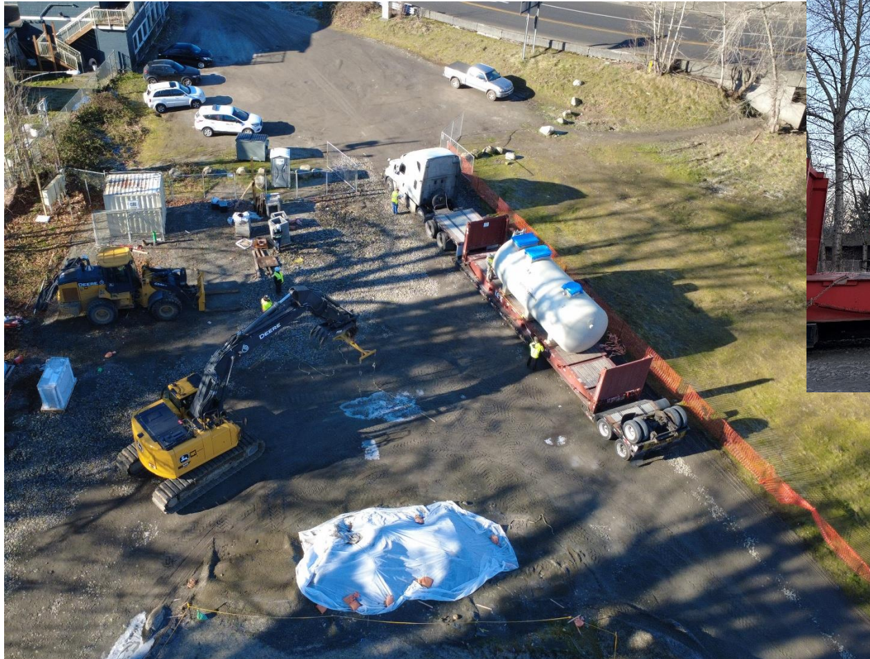
Delivery of 4 Kubota FRP tanks
