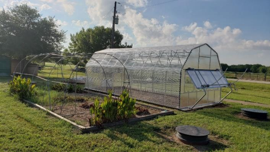
Wetland cells, one covered with the Greenhouse
