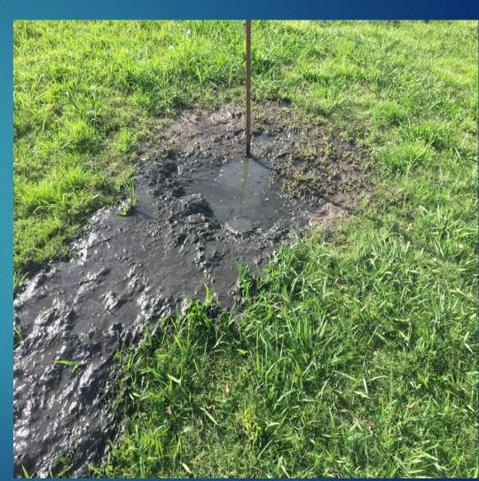
Overflowing septic tank caused by unknown/uncleaned filter.
