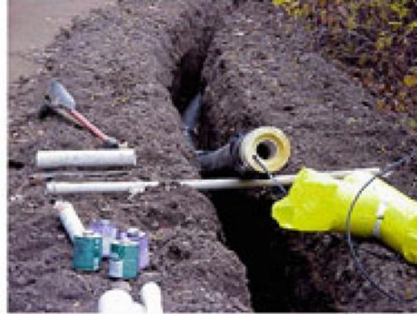
Trencher to dig 2-3 feet deep; insulated line for cold climates (on right).
