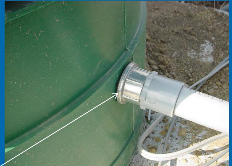
*Power to pump and float leads maintaining good watertight connections from the panel to the tank*
