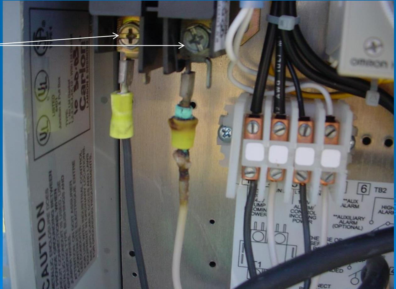
This is from the heat caused by the loose connection
