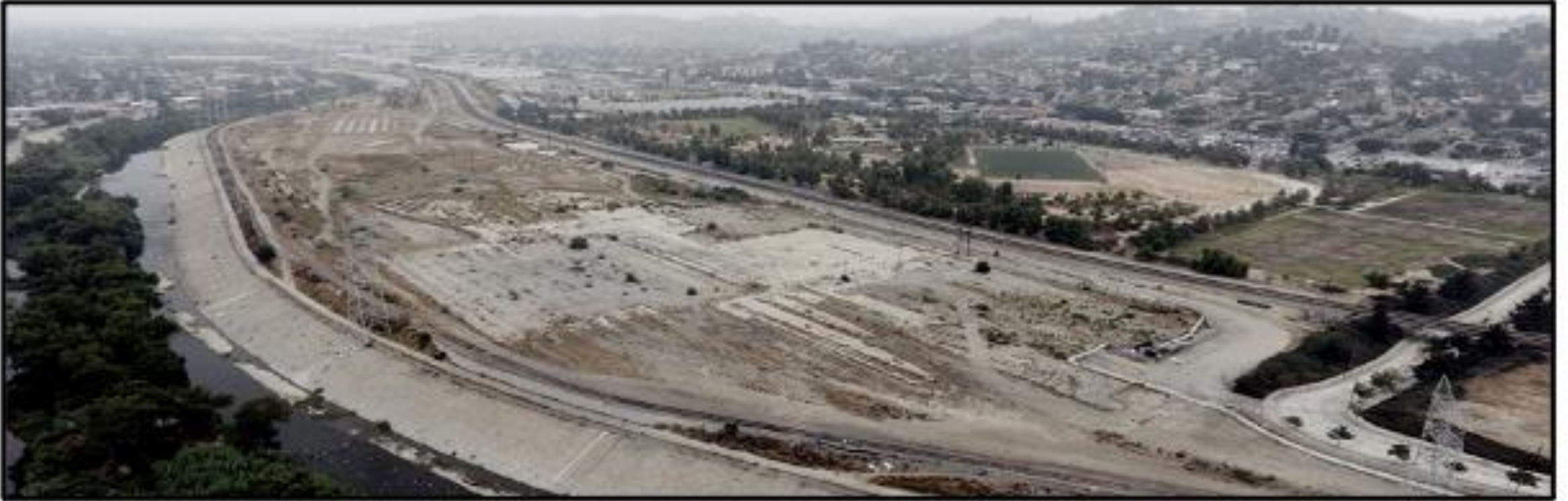
Taylor Yard, one of the study pilot locations, a former railyard on the LA river.
