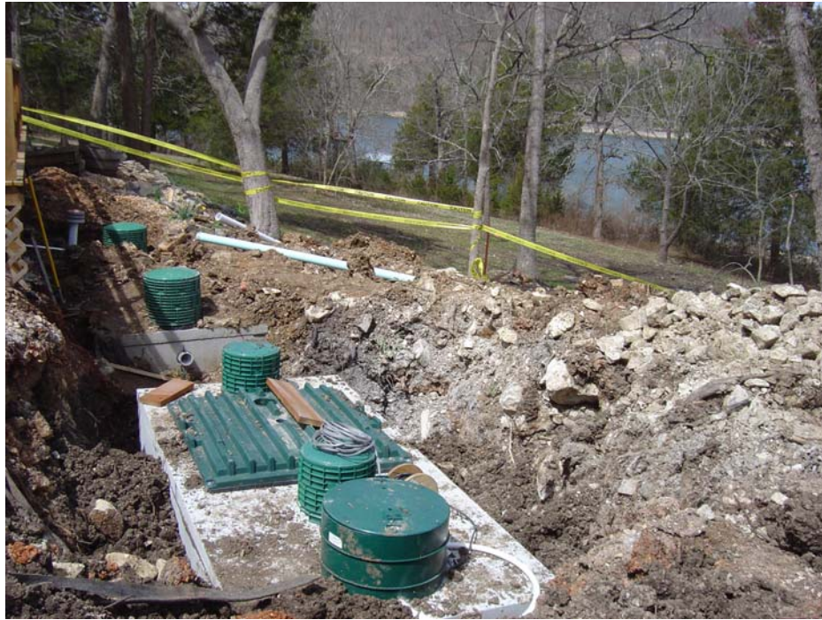
Figure 4 – Tank installation for a drip dispersal system
