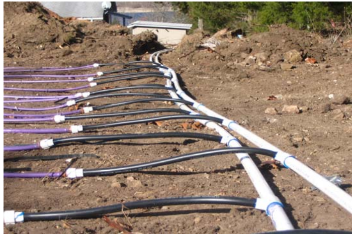
Figure 3 – Drip dispersal lines and return lines being installed
