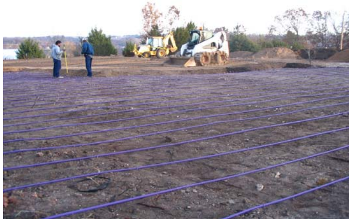
Figure 3 – Drip dispersal lines and return lines being installed
