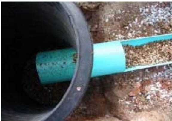
Figures 7 and 8 – 12-inch Lysimeter installation
