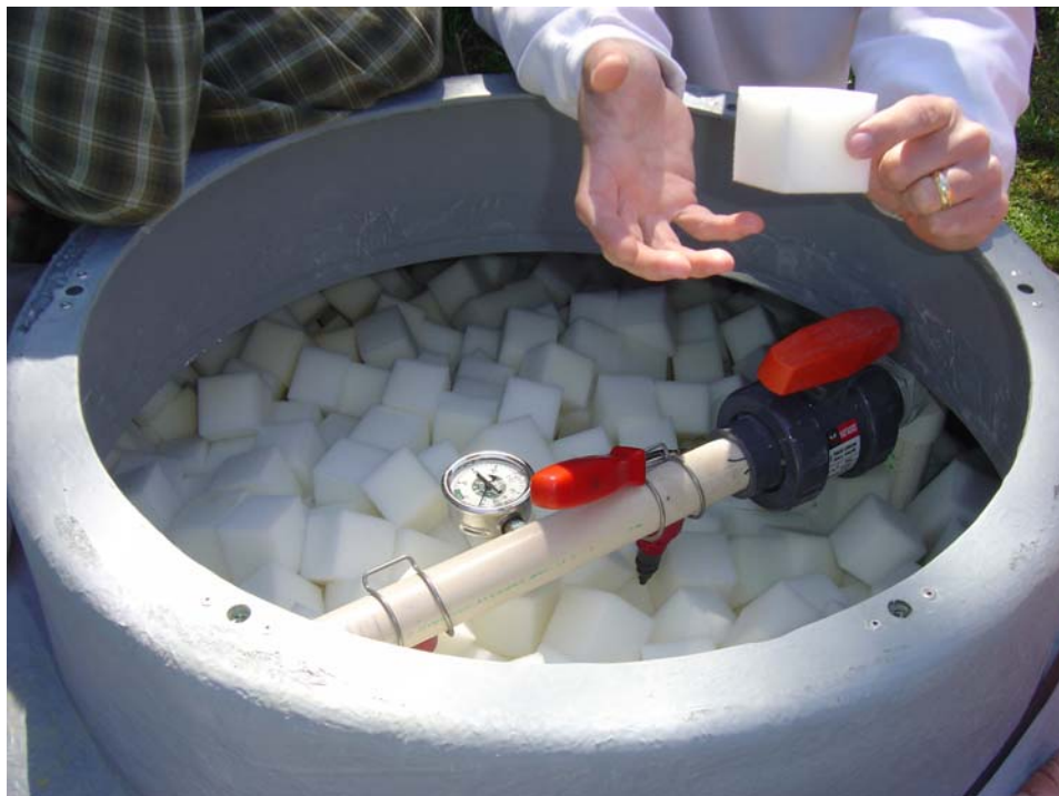
Figure 5 – Microbiotic biological reaction chamber media, foam cubes
