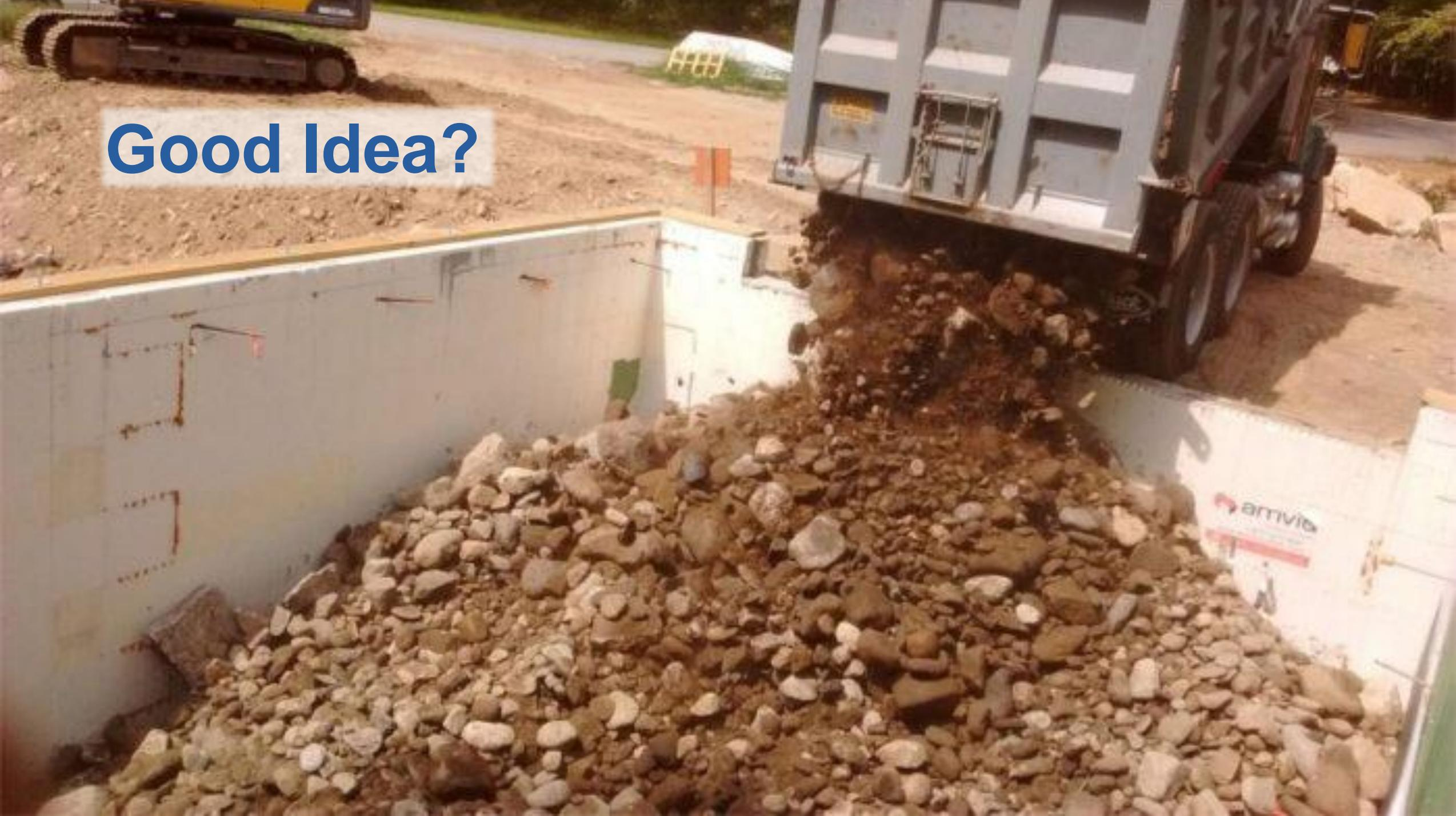
Will the skid steer load move the wall or retained soil?
