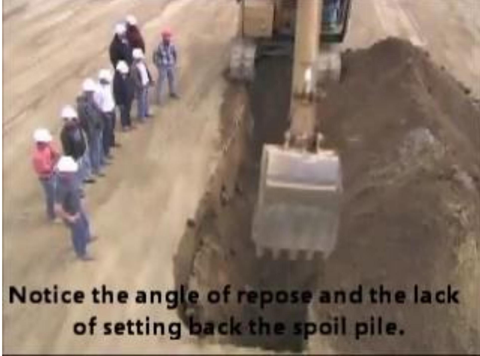
**Notice the angle of repose and the lack of setting back the spoil pile.**
