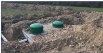
Image 37: Installation of an advanced treatment system. (Photo courtesy of Stone County Health Department)
