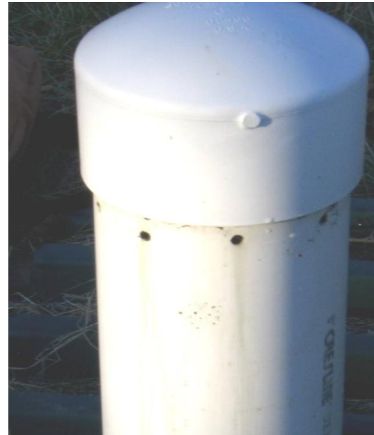
Inadequate Venting
