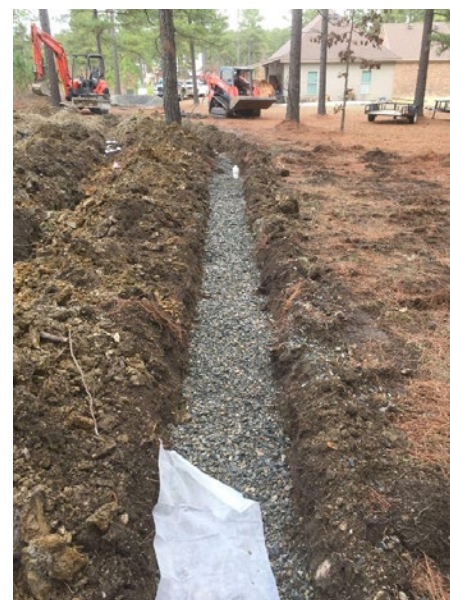
Figure 2: Example of a gravel-filled trench with low-pressure-distribution piping installed for uniform dispersal of treated effluent at each site with the infrastructure installed to monitor groundwater depth.
