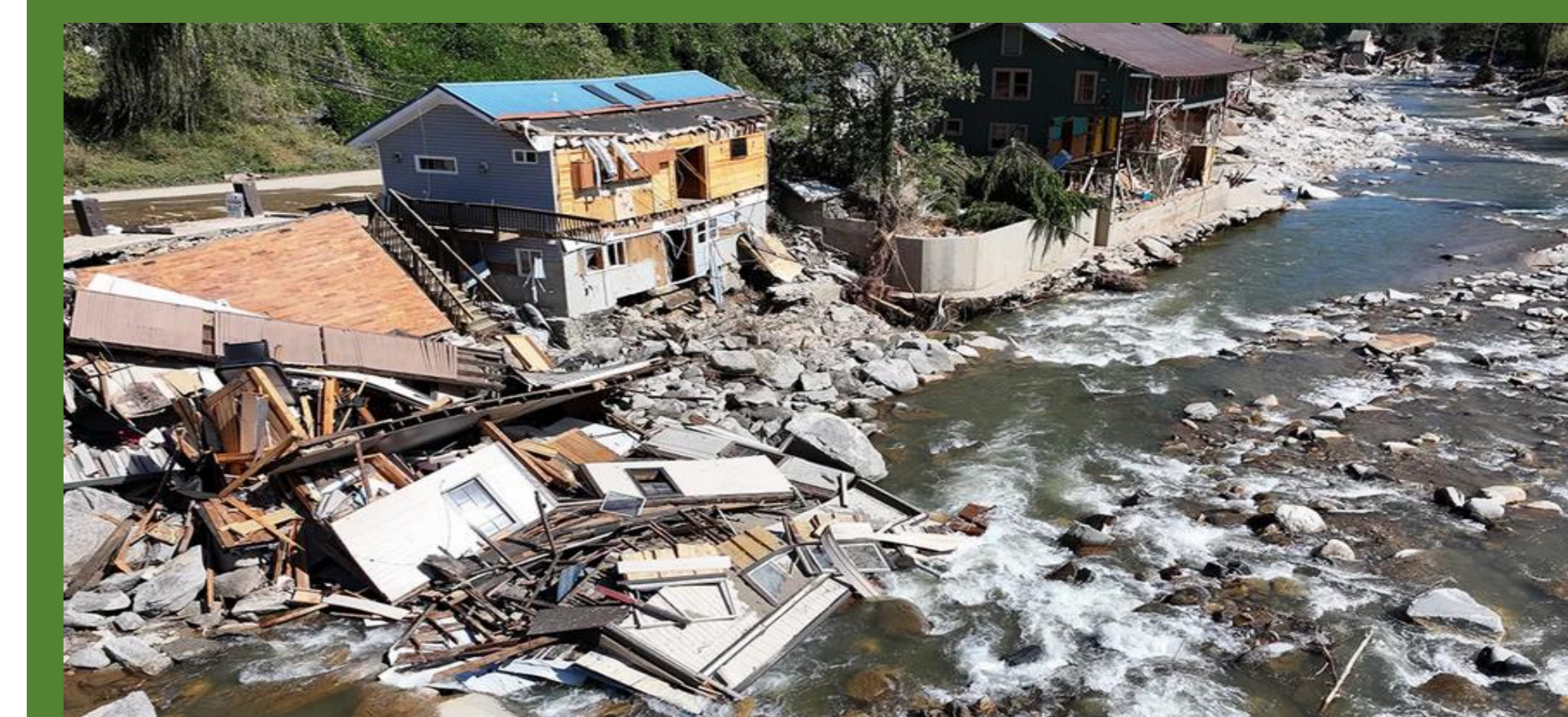
An aerial view of destroyed and damaged buildings in the aftermath of Hurricane Helene flooding on Oct. 8 in Bat Cave, N.C. (Mario Tama/Getty Images)
