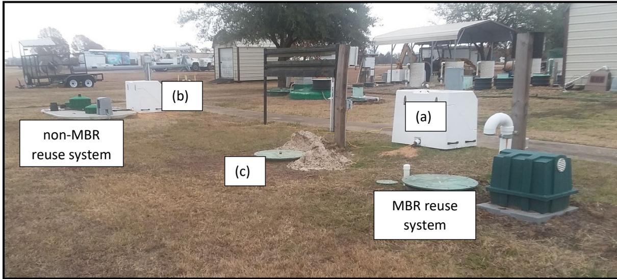
Figure 6: Field layout of the MBR and non-MBR reuse systems. (a) and (b) are the weather-proof boxes each housing two refrigerated composite samplers. (c) is ozone tank for MBR effluent.
