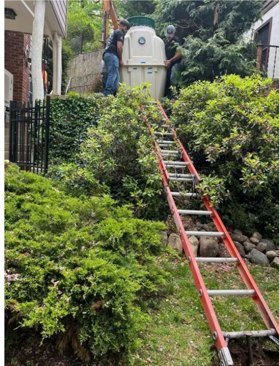
Figure 6. Installing a FujiClean Unit on Difficult to Access Site
