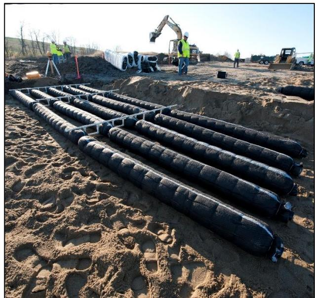
Fig. 2 Typical CTD system prior to backfilling with system sand and final grading
