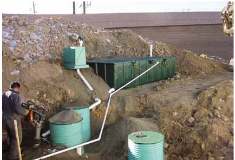
The installation of an AdvanTex Treatment System at the gas station/auto parts store, which is part of the field trip. Photo courtesy of SCG Enterprises, Inc.
