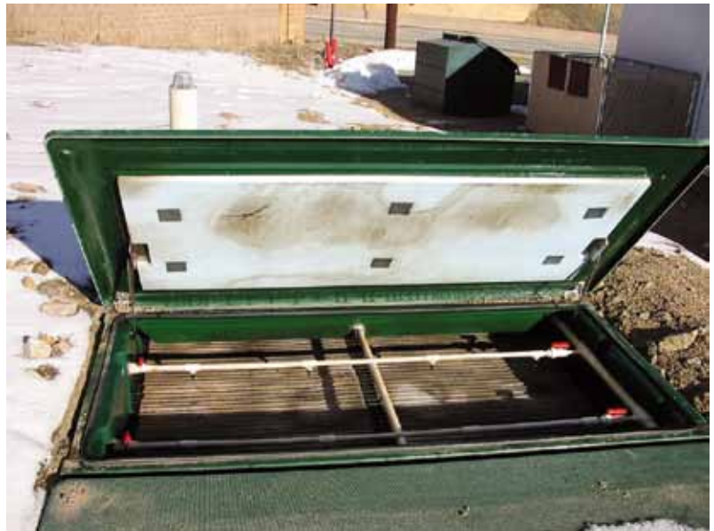
The media filter portion of the treatment system that will be visited on the field trip. Photo courtesy of SCG Enterprises, Inc.
