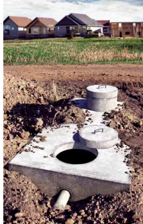
A precast concrete septic tank.
