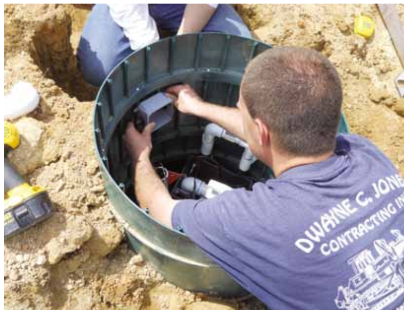
Jones Pump Service workers installing a Bionest nitrogen treatment unit.
