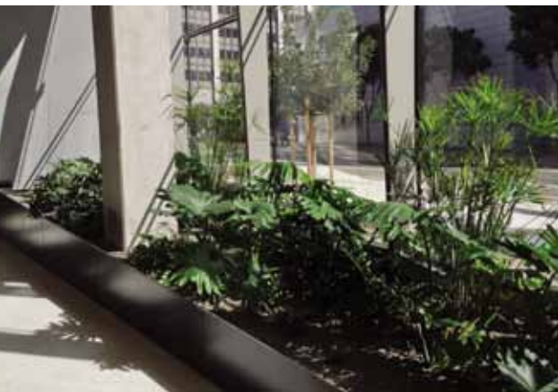
The Living Machine uses plants to treat all of the building's wastewater in the lobby and surrounding sidewalk. All photos in this layout provided by the San Francisco Public Utilities Commission.
