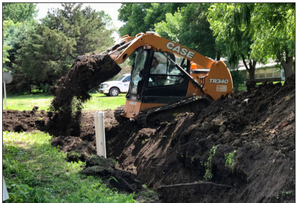
Backfilling the Rowan project
