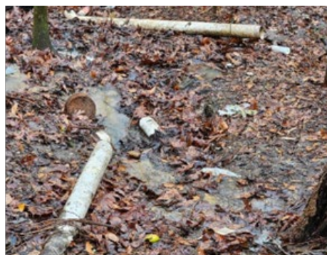
Photo 2. Examples of straight pipes and failing septic systems in the Black Belt Region of Alabama.
