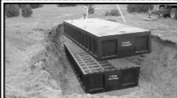
18,000 Gallon Precast Concrete Tank
