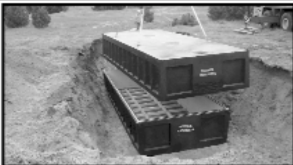
18,000 Gallon Precast Concrete Tank
