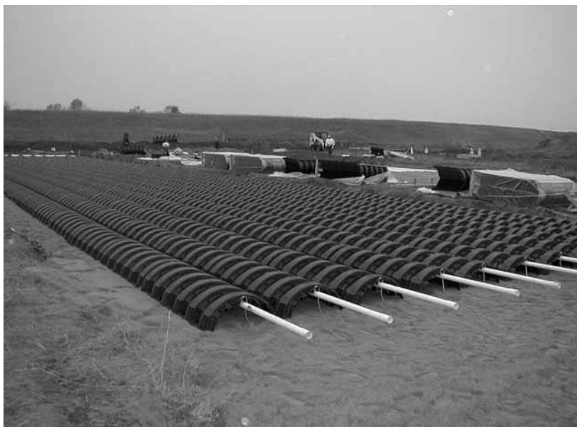
Installation of infiltration beds for soil disposal of treated wastewater. Infiltrator ® chambers, each enclosing a pressure distribution lateral, are placed parallel to each other on a sand bed and then covered with native soil. Copyright © 2006, North American Wetland Engineering, LLC.
