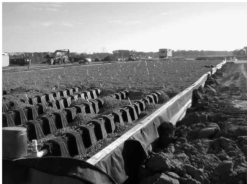
Installation of an engineered wetland wastewater treatment system: a recirculating gravel filter for treatment of domestic wastewater. Copyright © 2006, North American Wetland Engineering, LLC.
