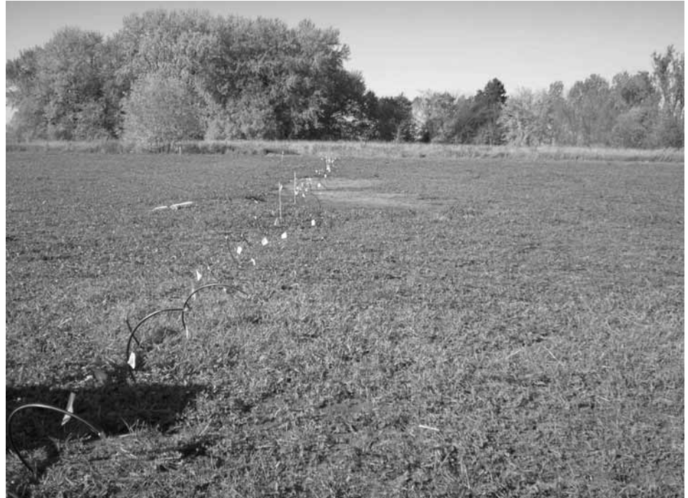
Drip irrigation disposal system following installation. Drip tubing is installed below grade using a vibratory plow or trenching device. Copyright © 2006, North American Wetland Engineering, LLC.
