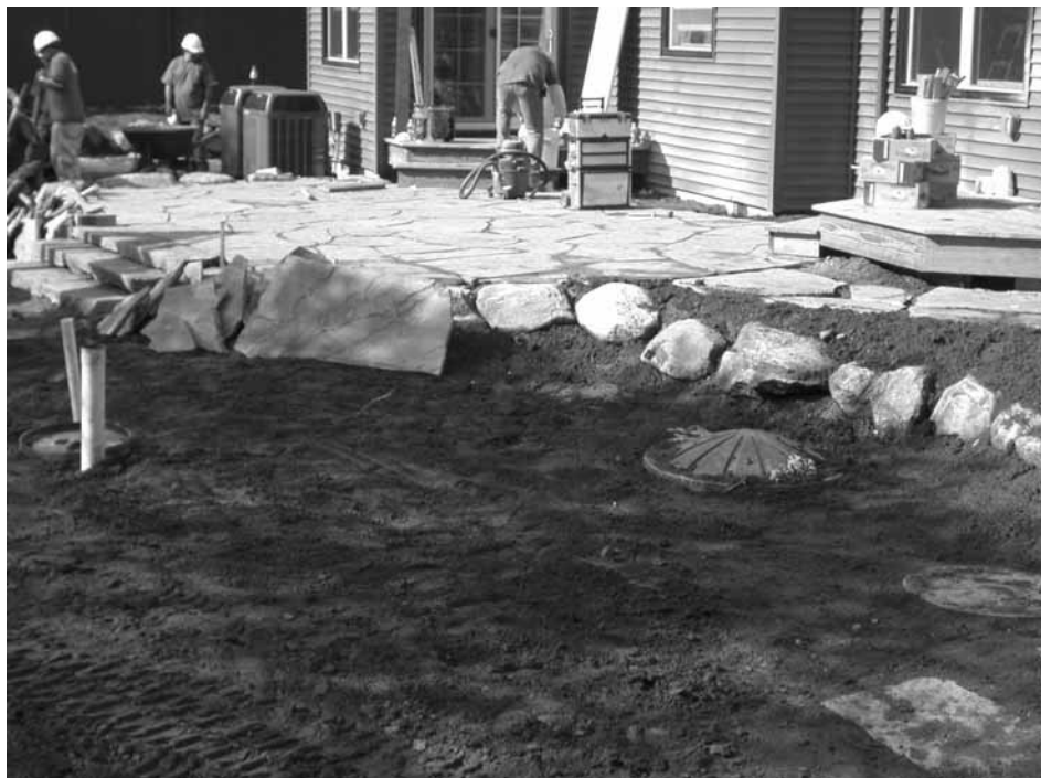
Access to the distribution box (left), aerobic pretreatment system (center back) and the septic tank (right) is worked into the landscape so that appropriate plantings will minimize their visibility.
