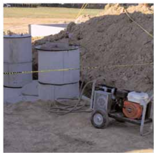
Testing in the field.
