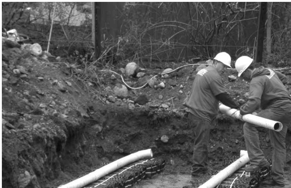
Eljen A42 GSF leachfield modules are placed on the sand on five-foot centers. Jeff Houser, engineer on the project, cuts solid pipe to form a closed loop at the end of the lines with assistance from Mark Eliassen, contractor.
