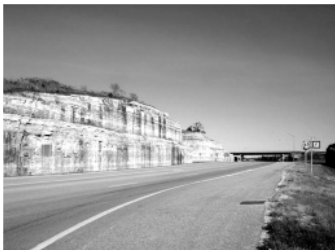
Road construction reveals how little soil there is around Table Rock Lake.
