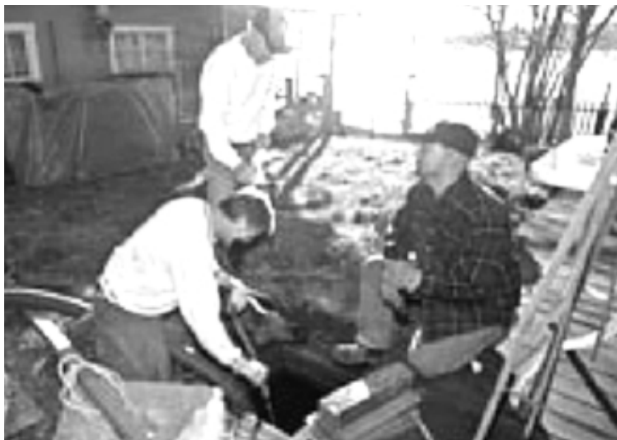
Donald McDonald of Seattle holds a light for Leon Borst, left, and Thad Bamford of AAA Septic and Pumping as they clean and inspect a decades-old septic system at his home on the Hood Canal near Tahuya.
