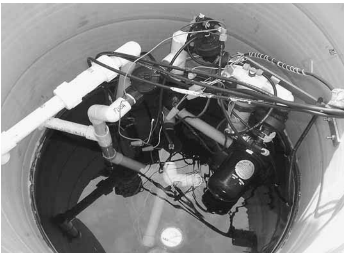
Fig. 8. Riser for a pump chamber where the drip distribution headworks was installed. The headworks must be removed before the pump can be pulled to be cleaned or replaced. The pump is housed in the vertical pipe located in the upper right of the figure. Obviously there is a problem with this system because the water is higher than normal.
