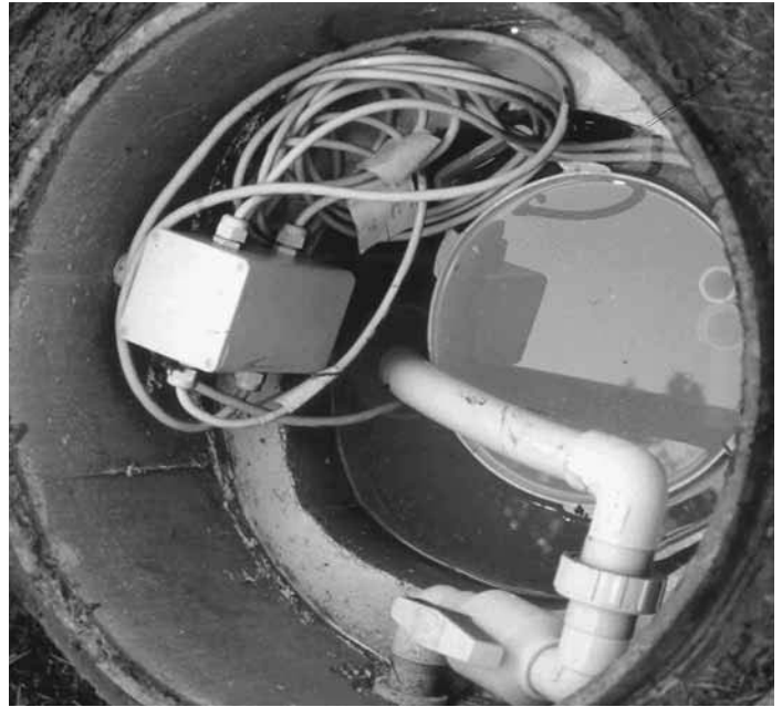
Fig.11. Construction debris in pump chamber from new home. Water is milky due to paint. Edge of valve handle is white, which should be black in the picture as is the side of the handle. (Picture by Dan Bush)
