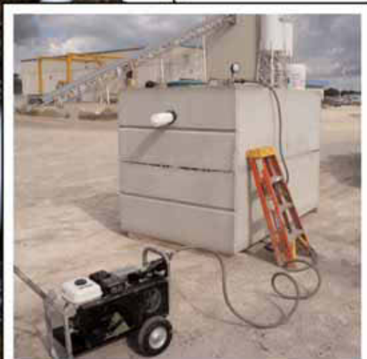
Testing at the plant.
