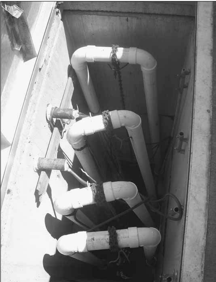
Fig. 4. A pump chamber using goose necks for each pump. In this case no easy disconnect such as a union was used. When the pump needs to be replaced, the horizontal pipe is cut and the pump is lifted out with the chain in this case.
