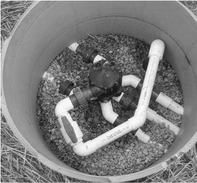
Fig. 10. Flexible PVC piping would make it easier to change out this distributive valve.
