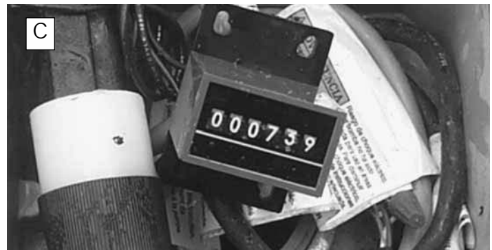
Fig. 1. Water meter, event counter and elapsed time meter (A). Water meter measuring flow to a drip field (B). Event counter in junction box measuring pumping events in a pump system (C). Event counter and elapsed time meter in control panel (D).
